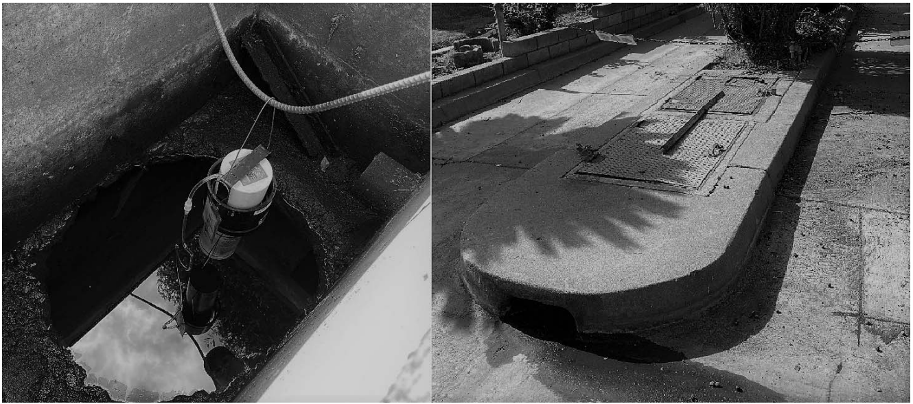
Figure 2. —The drain and two access lids to the double chambered BMP on Nada St. in the City of Downey (right). The drip system hanging in the inundated dry well (left).
