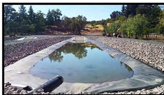
Figure 7. —One of the \frac{1}{4} -acre ponds partially filled to demonstrate the contoured bottom. Other features include a concrete ramp at the end and rip rap rocks around the perimeter.
