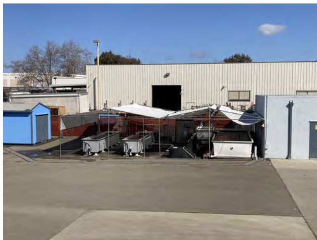
Figure 1. —Outdated outdoor fish storage structure that was demolished to make space for an indoor fish rearing facility.
