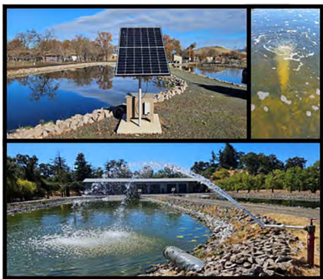
Figure 9. —(A, B) Solar aeration units pump fresh oxygen into our pond systems from the bottom. (C) PVC elbows have been added to our water mains to eject and aerate all new water entering the ponds. Both of these systems provide ample oxygen into our pond systems to maintain our fish and muck-eating microorganisms.
