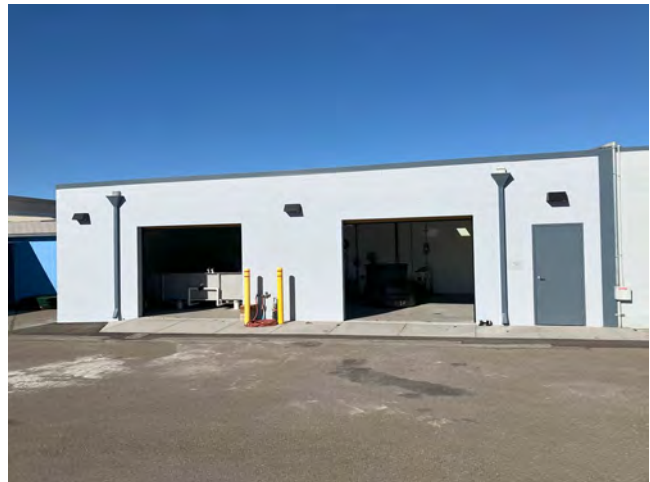
Figure 2. —Exterior of the new, 1,115 sq/ft indoor Aquaculture Facility for rearing fish year-round.
