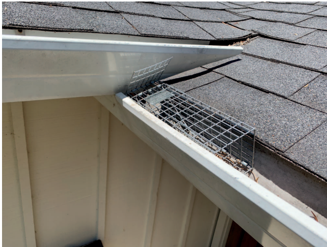
Figure 1. —Caption: One-way door installed in a gutter to remove a red fox squirrel from an attic area. Photo by Kimberly Daum, ACVCSD.
