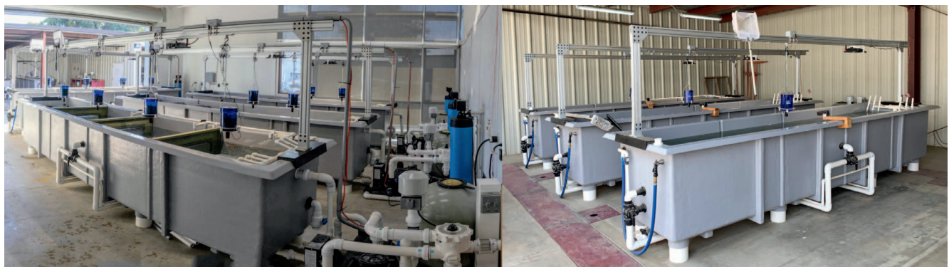
Figure 4. —The installed automatic feeder system in the indoor and outdoor mosquitofish facility.
