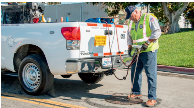
Figure 4. —Inspector from the Orange County Mosquito and Vector Control District applying anEPA-approved, larvicidal spray through a drop inlet hole to the USDS.
