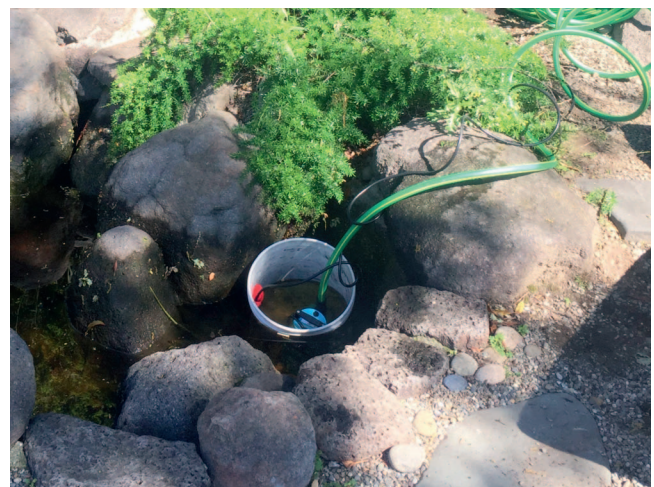
Figure 2.—Use of a sump pump and hose to drain a deep pond. Bucket with screened ports serves to prevent debris from clogging the pump.
