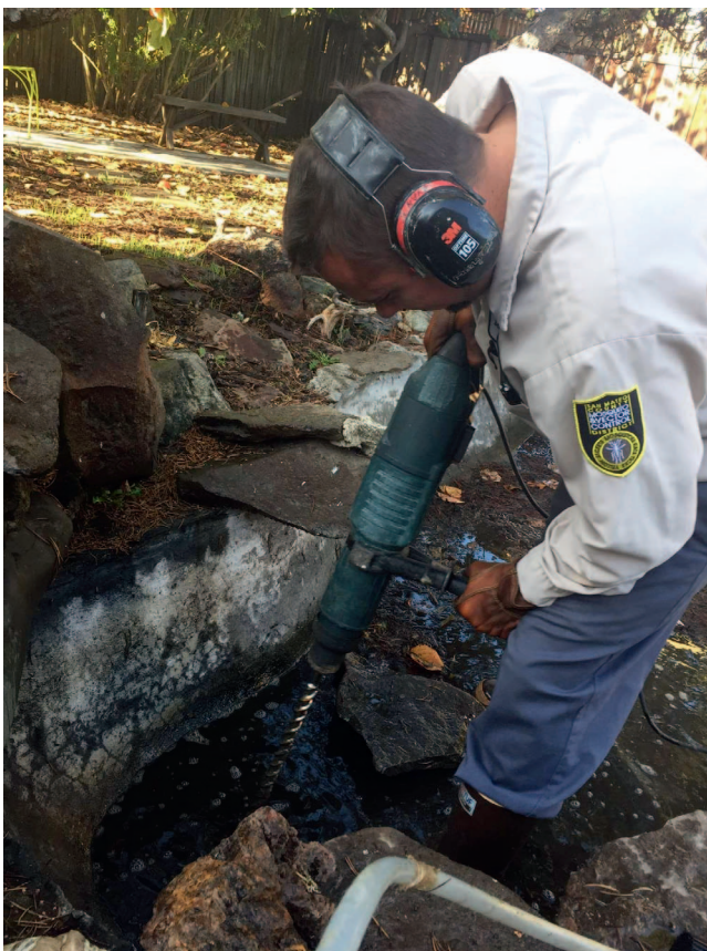
Figure 4. —Technician using an impact drill to provide drainage to ensure the pond will no longer hold water.
