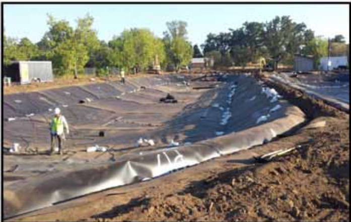
Figure 3: The 8mm plastic liner installation and welding process.
