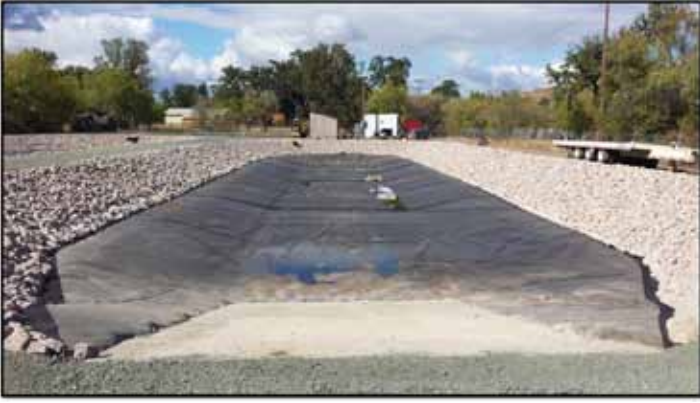
Figure 5: A completed pond showing all the features of this pond design.
