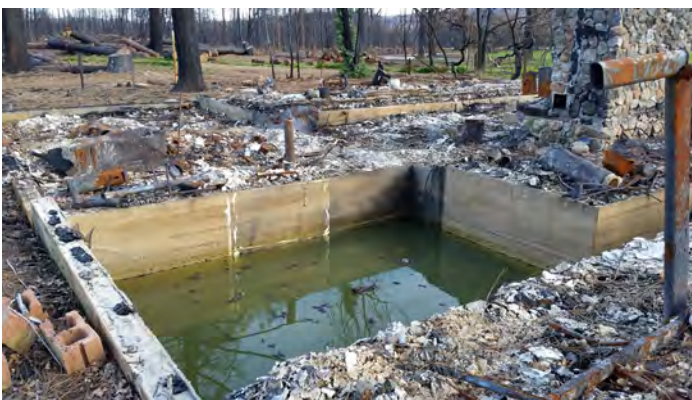
Figure 5. A basement holding water is all that remains of this house.
