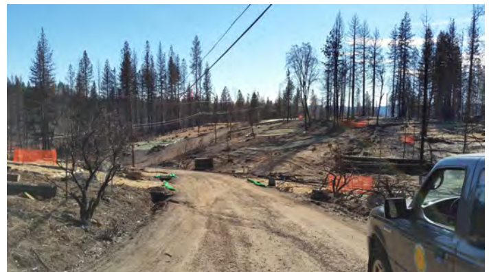
Figure 7. The same neighborhood in Cobb after cleanup was complete. Orange construction fences surround damaged septic tanks and other holes in the ground.
