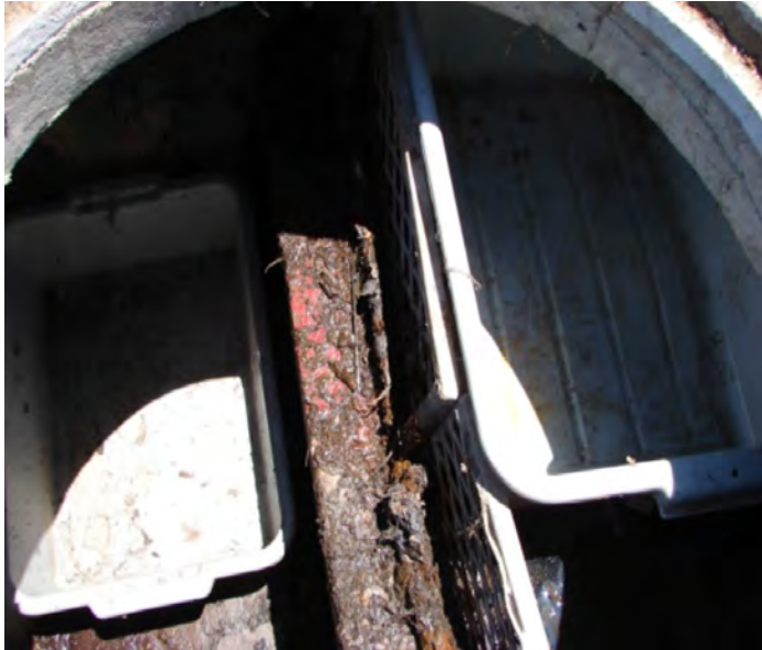
Figure 3. Trays used to collect debris inside the catch basins.
