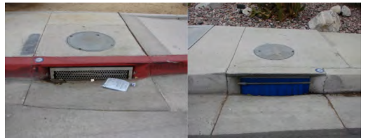
Figure 2. Left: Automatic retractable screen (SS). Right: Baleen bristle screen (BB) (2/27/2014).
