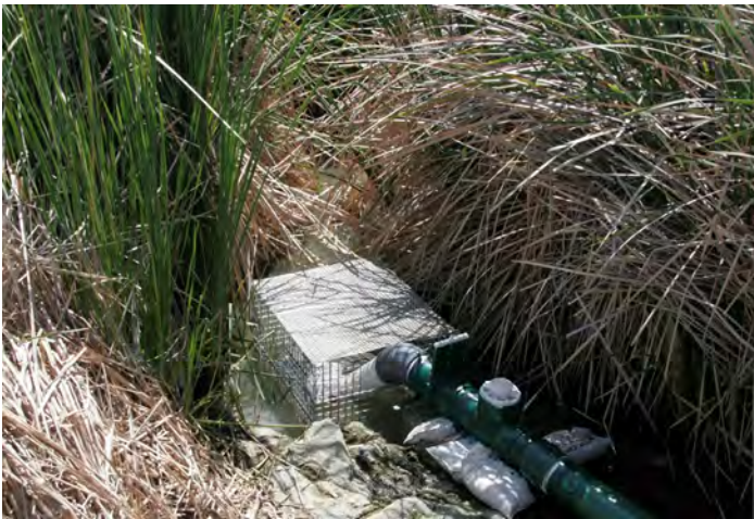
Figure 1. Photograph of water management siphon intake pipe and valve at the west side of the Big Canyon Pond. The intake pipe is housed in a stainless steel cage to prevent debris accumulation and clogging.
